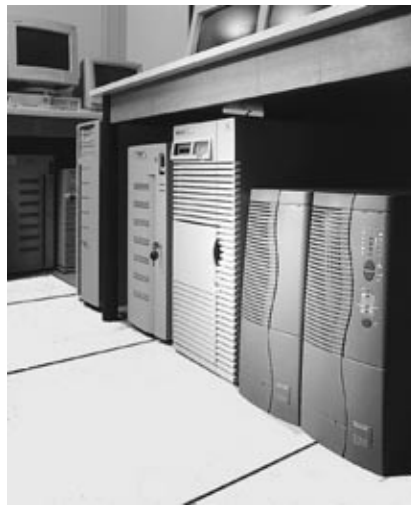
Fig. N30b : UPS unit achieving disponibility and quality of computer system power supply
