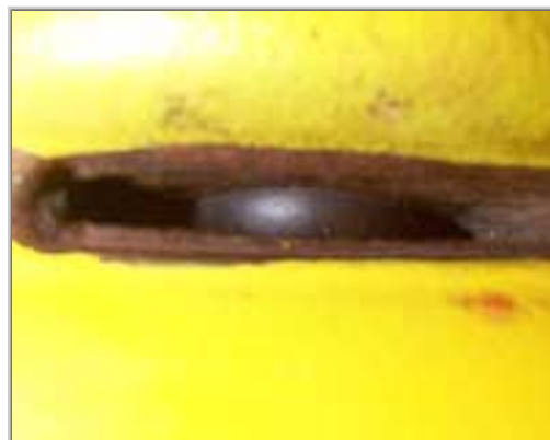
Installed expandable plug visible through the block weep hole.
