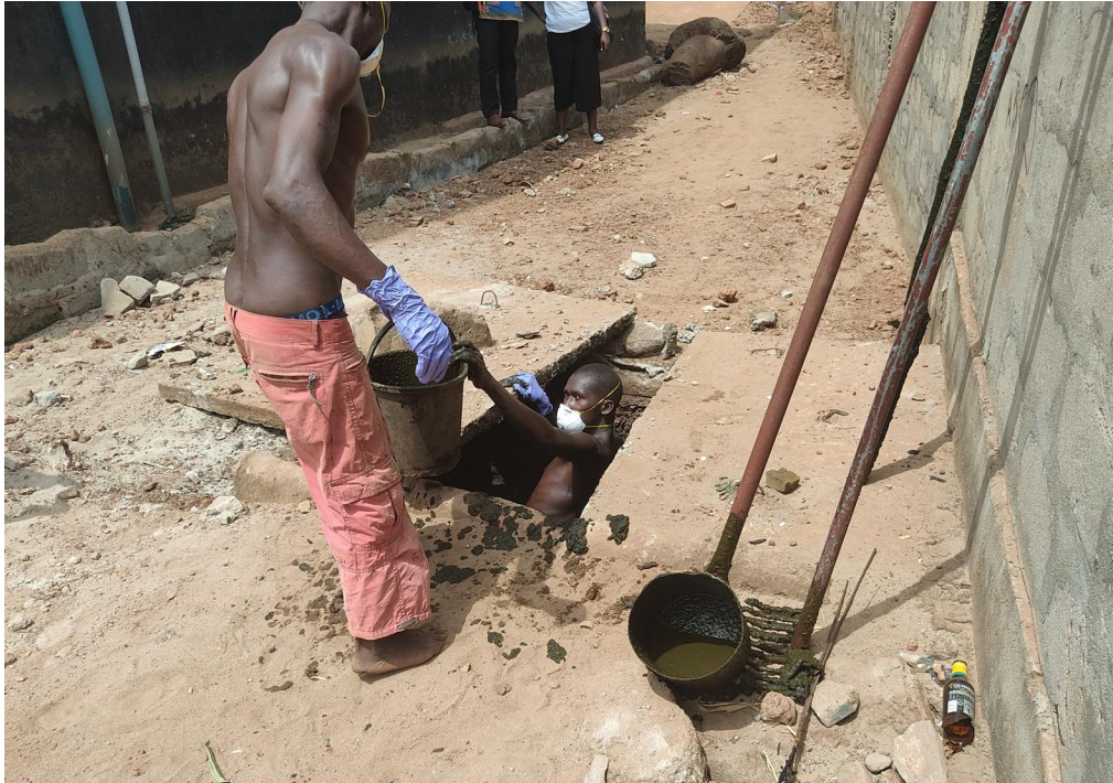
Fig. 6: Manual pit emptiers at work in Freetown. Photo: N. Leblond.*
