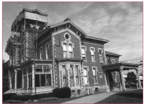
Kalamazoo, Michigan American Red Cross Restoration Project
