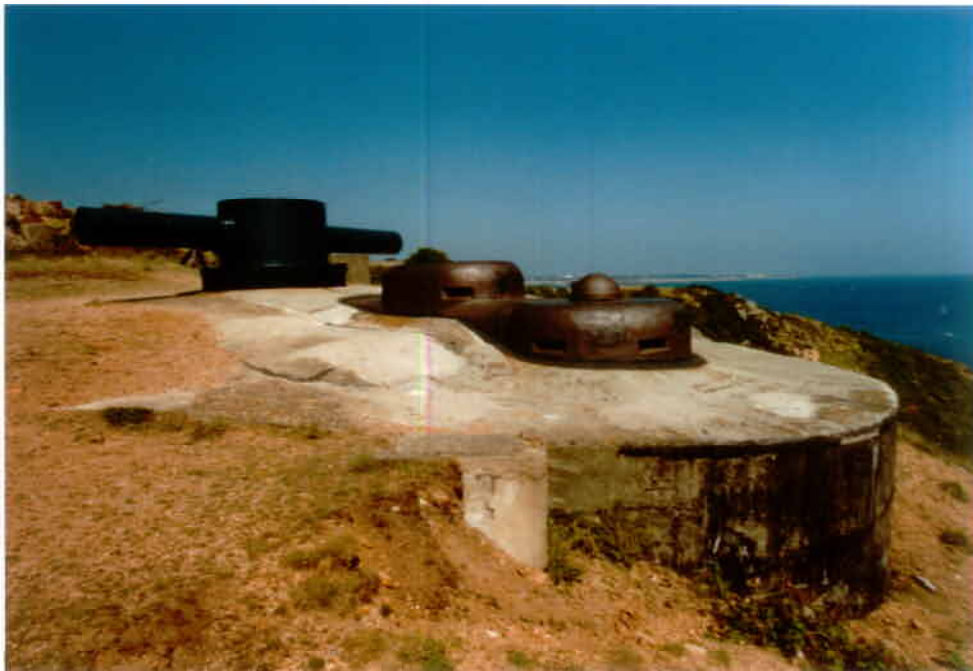
The steel domes of the M132.
