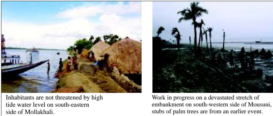
Photo 4.1: Embankments in field study islands
